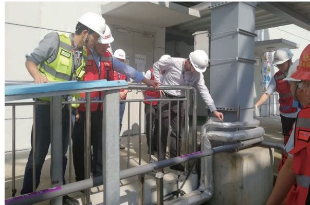
Scene of safety inspection
