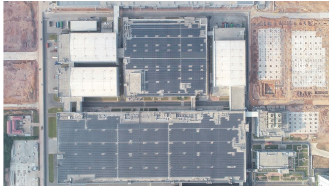
Aerial Photography of TCL Huizhou CSOT Photovoltaic Power Generation
