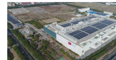
Rooftop PV Solar Systems at Suzhou CSOT
